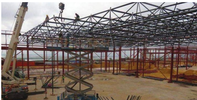
◀ Erection of roofing assemblies.
